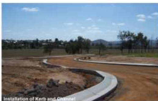
Installation of Kerb and Channel
