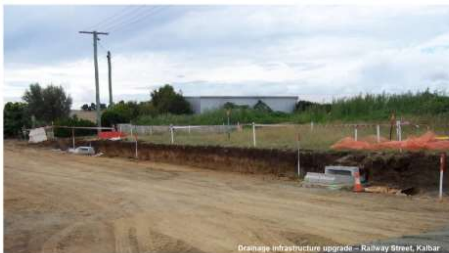
Drainage infrastructure upgrade – Railway Street, Kalbar
