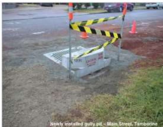
Newly installed gully pit - Main Street, Tamborine
