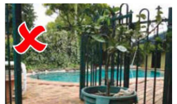
A pot plant could prop open a gate or be used to climb into the pool area and must be removed.
