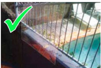
A flat polycarbonate sheet can be used to shield a climbable object.
