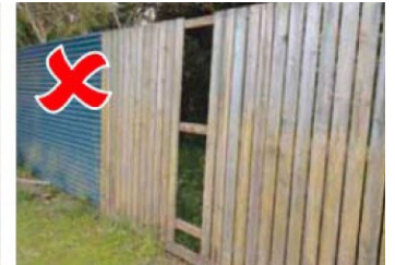
Gaps in a fence over 100 millimetres can provide easy access.
