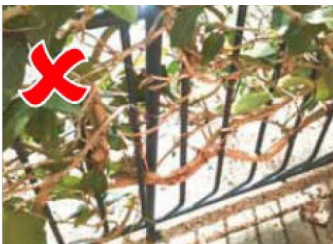
Remove any vegetation that can be used to climb into the pool area.
