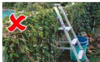
A ladder is a climbable object and must be removed. The vegetation shown is acceptable as it is not climbable.
