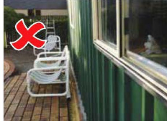
Windows that provide easy access to the pool area must be fixed permanently closed.
