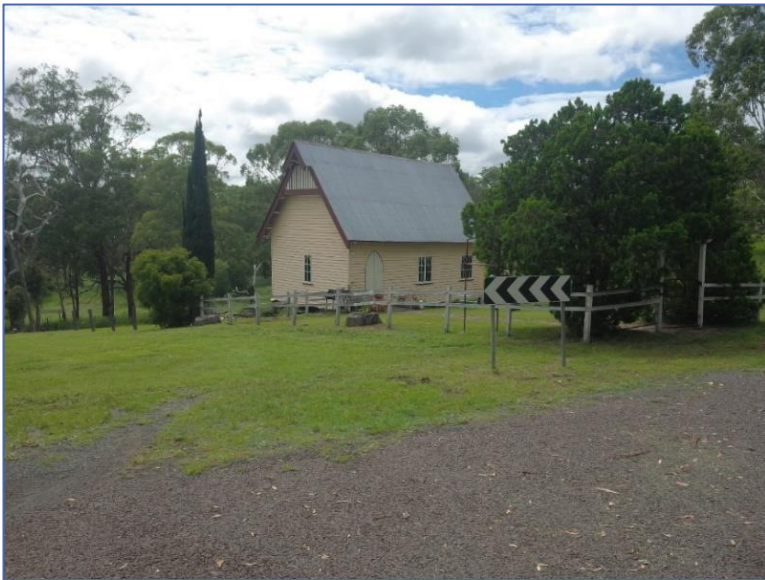
Figure 1: The former St Andrew's Anglican Church, Maroon is now used as a private residence
