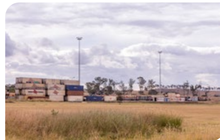
SCT Intermodal Estate, Bromelton State Development Area
