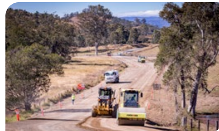
Roadworks at Kooralbyn
