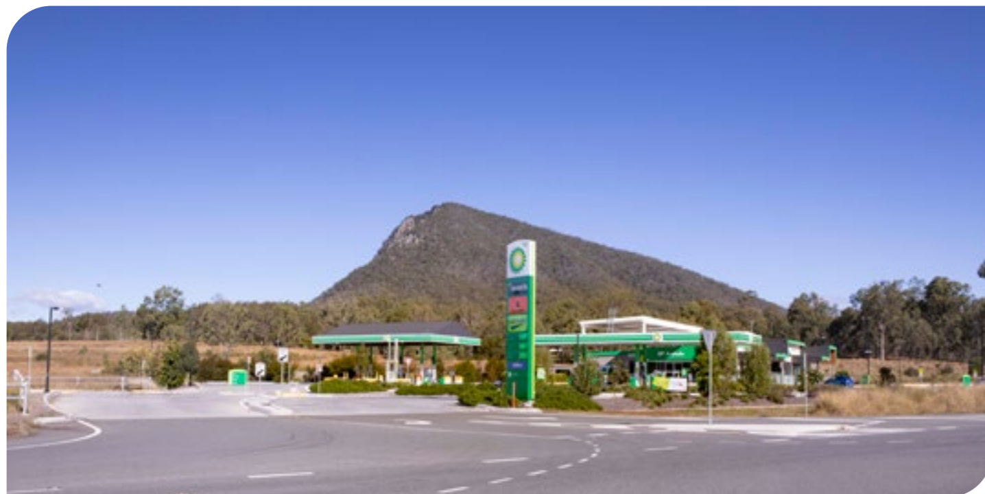
BP Service Station, Aratula.
