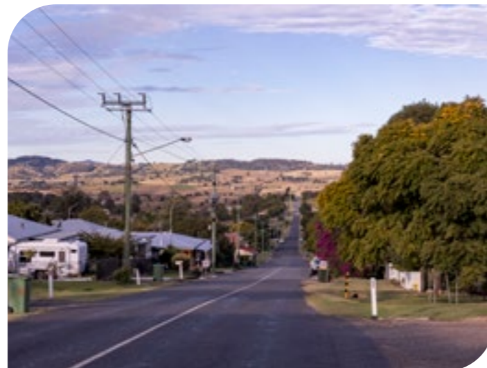
Roadvale Road, Roadvale
