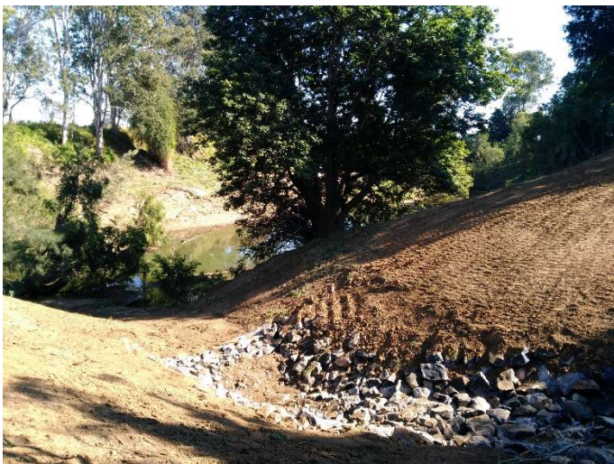
Figure 3: Gully stabilisation beside the Logan River
