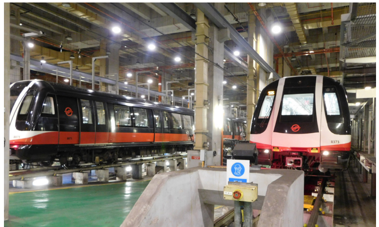
World's largest underground train depot (SMRT)
