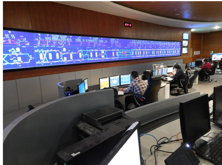
SMRT control centre for automated train operation
