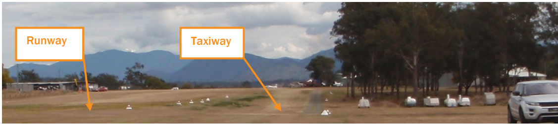
Figure 9 Taxiway – facing southwest
