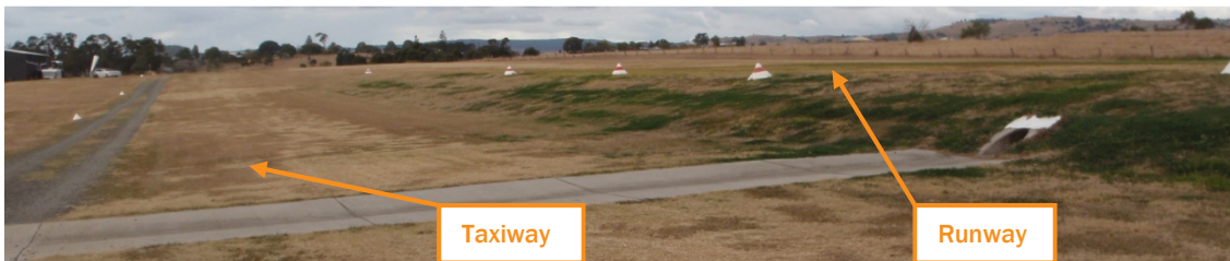
Figure 10 Taxiway - facing northeast
