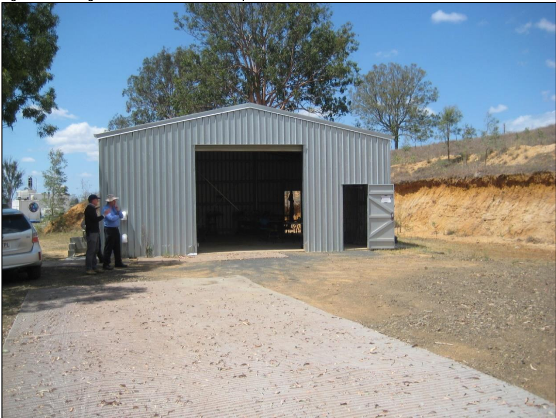
Figure 5: Existing shed to be utilised as the operations centre
