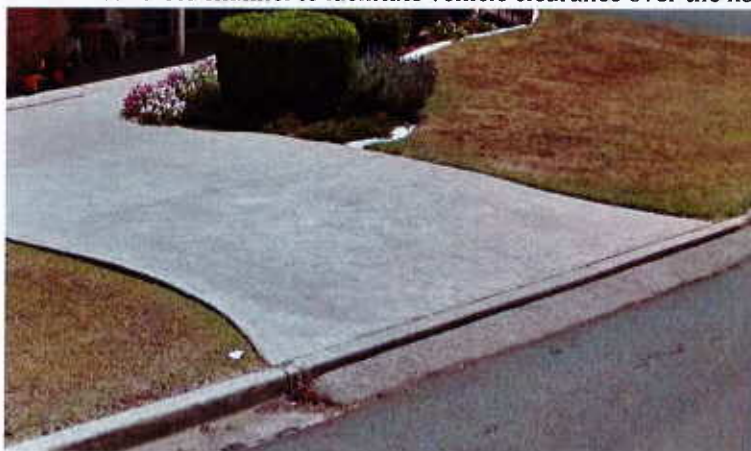
Figure 2-11 Driveway at 1 Valleyview Drive
