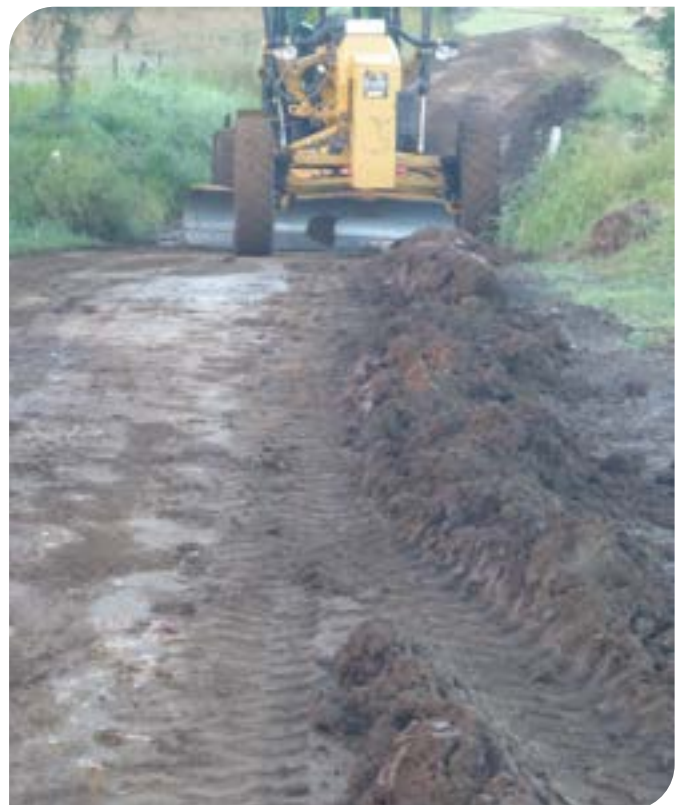
Kerry Creek Road holding works.
