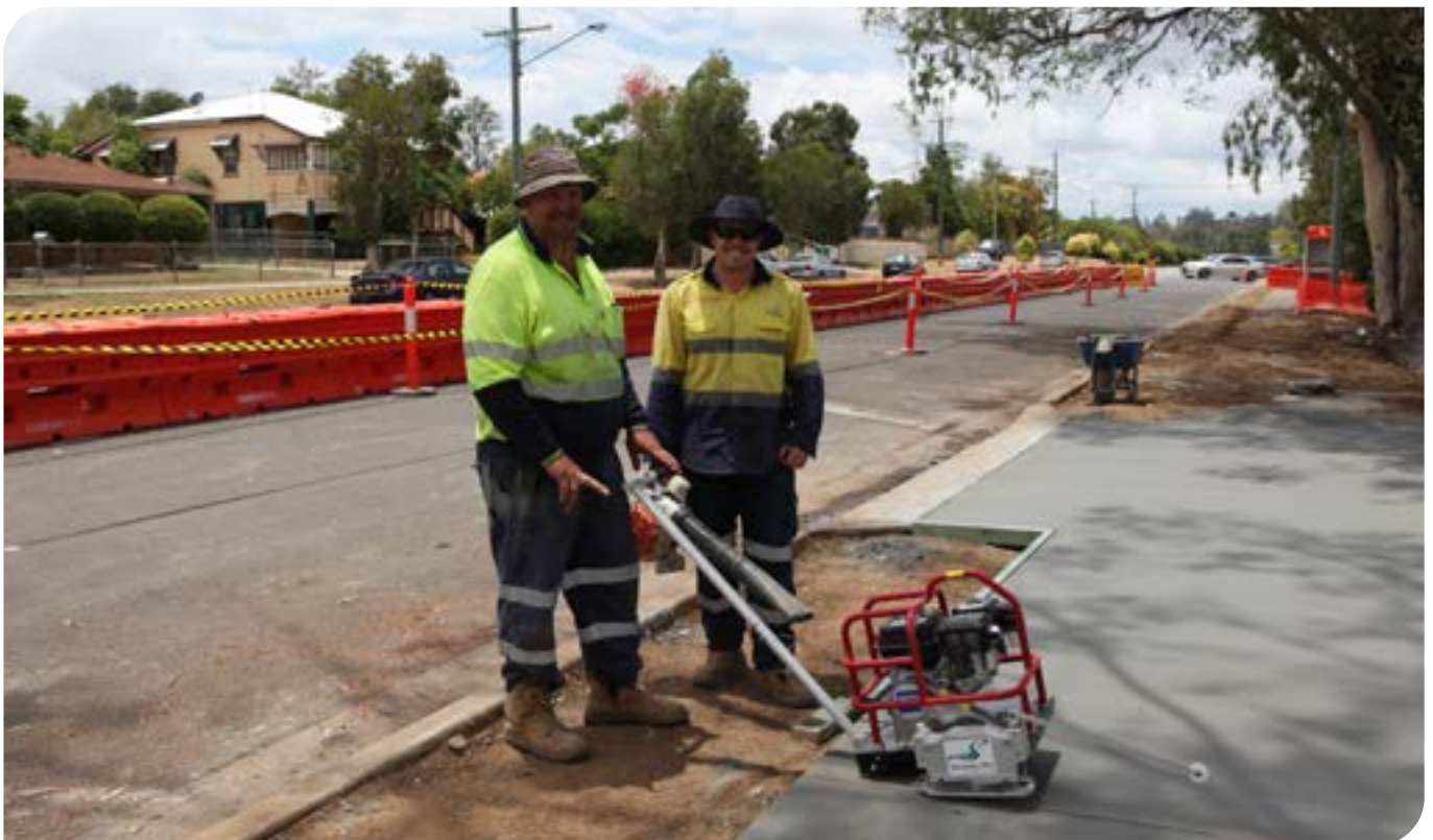
Scenic Rim Regional Council employees at footpath reconstruction site in Beaudesert.
